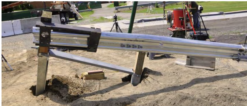
Figure 309. Post-test photo of Test 14001M for 2-inch reduced embedment case.
