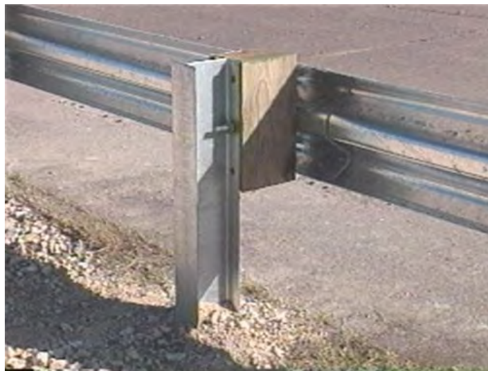
Figure 1. Modified G4(1S) with wood blockouts.[Bullard96]
