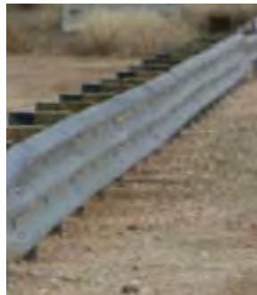
Figure 21. Photo of the thrie-beam guardrail with routed wood blockouts. [ Bullard10 ]
