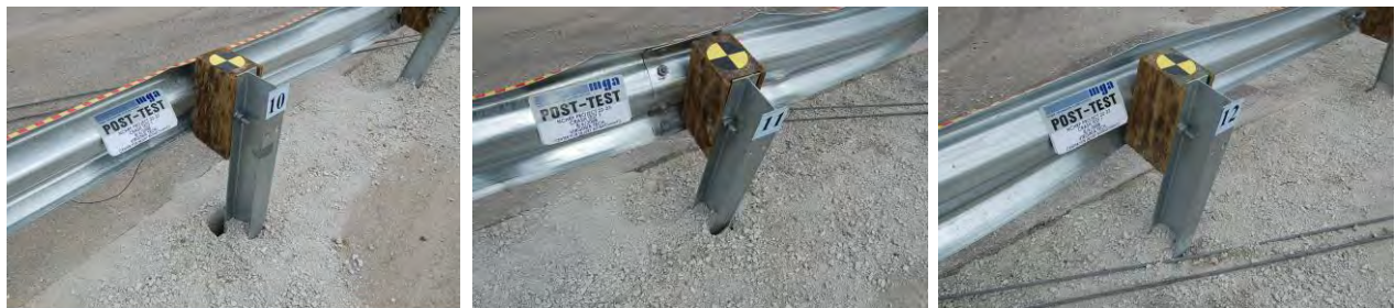
Figure 29. Guardrail damage in Test C08C3-027.1. [Fleck08]
