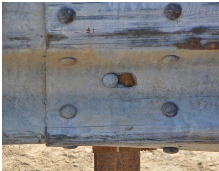
Figure 340. Typical mounting position for post-bolt was on the downstream side of the slotted hole on the rail.
