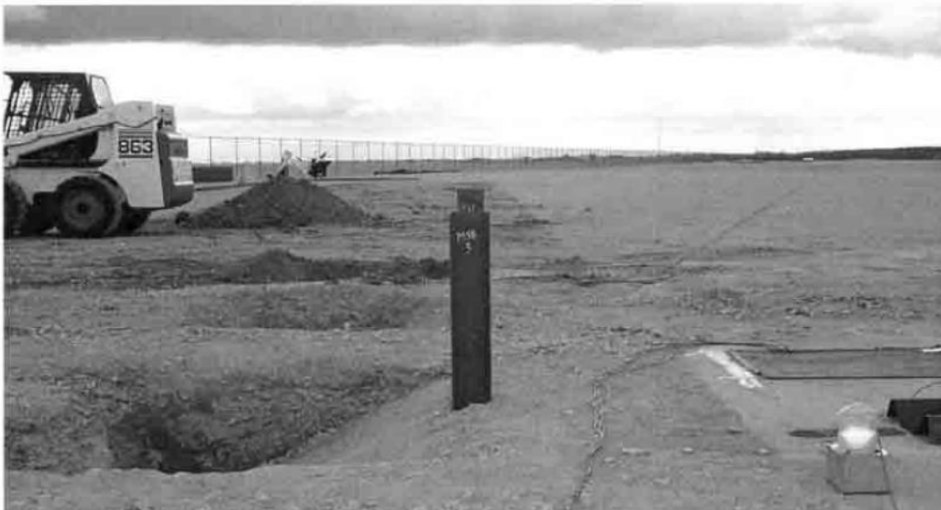
Figure 36. Typical steel post test installation for bogie impact testing. [Polivka00b]
