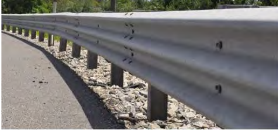
Figure 17. Photo of the standard three-beam guardrail (G9; SGR09a)
