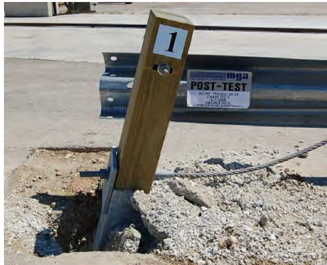
Figure 62. Post-test photo for Test MGA C08C3-027.2 showing the excessive anchor movement that occurred during the test.[Fleck08b]
