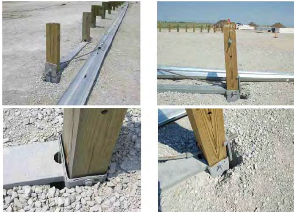
Figure 202. System damage at upstream anchor resulting from Test MGSDF-1.[Hascall07]
