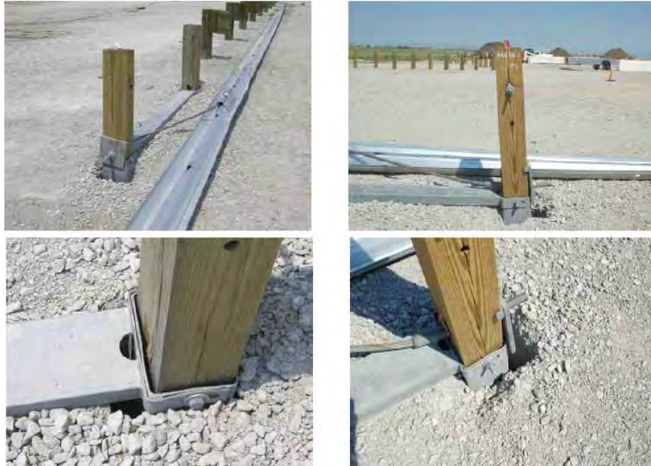
Figure 185. Damage to end-terminal anchor in full-scale crash Test MGSDF-1.[Hascal07]
