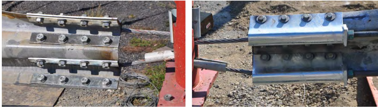
Figure 338. Anchoring of the downstream end of the rail for Test Series 14004.
