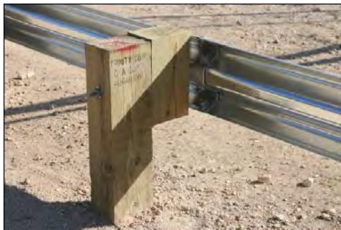
Figure 9. Photo of the G4(2W) guardrail Test 476460-1-5 test installation.[ Bullard10 ]
