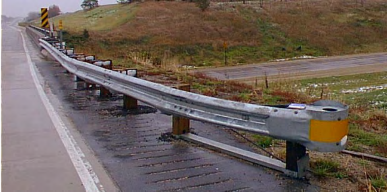
Figure 31. Modified Eccentric Loader Breakaway Cable Terminal. [Patzner99]
