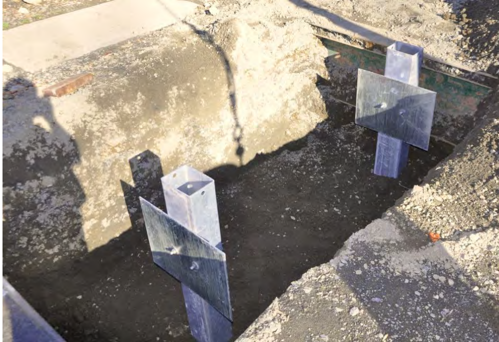
Figure 178. Photograph of anchor tubes with soil plates during installation.
