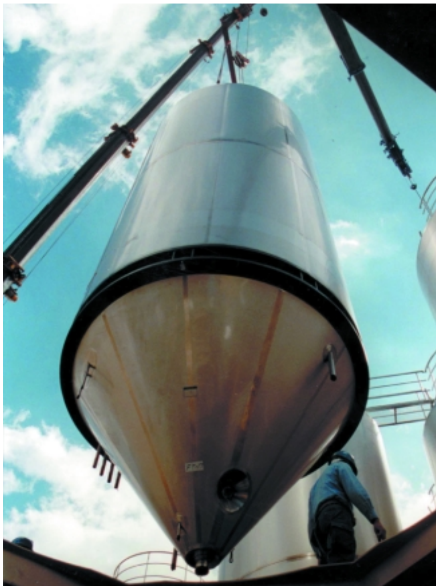
■ Figure 1. Installation of a batch, 765-bbl beer fermenter made of stainless steel. (Courtesy of Paul Mueller Co.)
