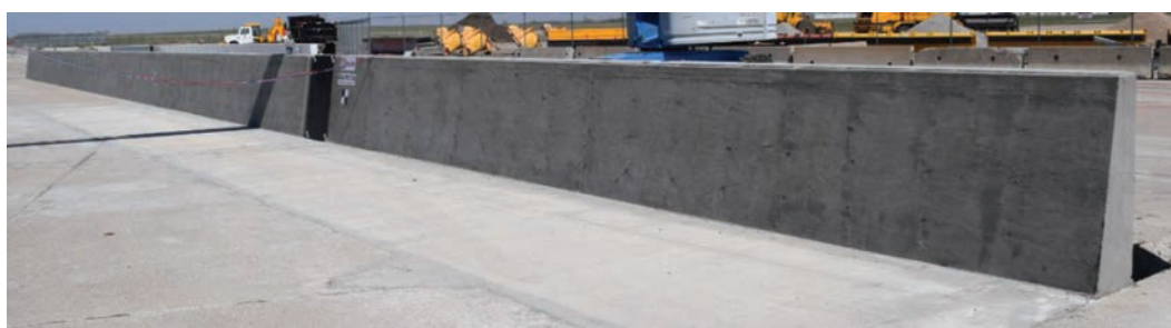
Figure 26. Test installation for Test MAN-1 [Rosenbaugh 2016].
