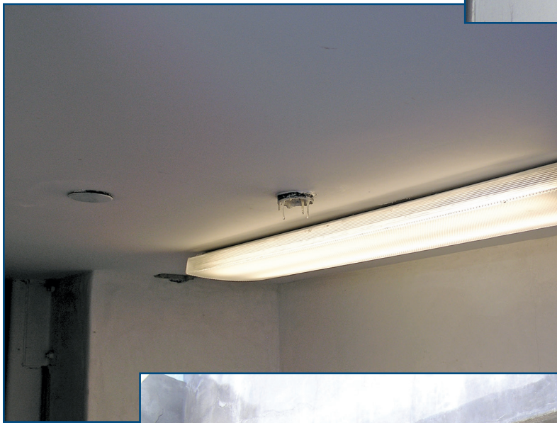
Figure 12 - Water leaking through residence utilities. Note the formation of stalactites from chronic leakage. The swimming pool is directly above this finished living space.
