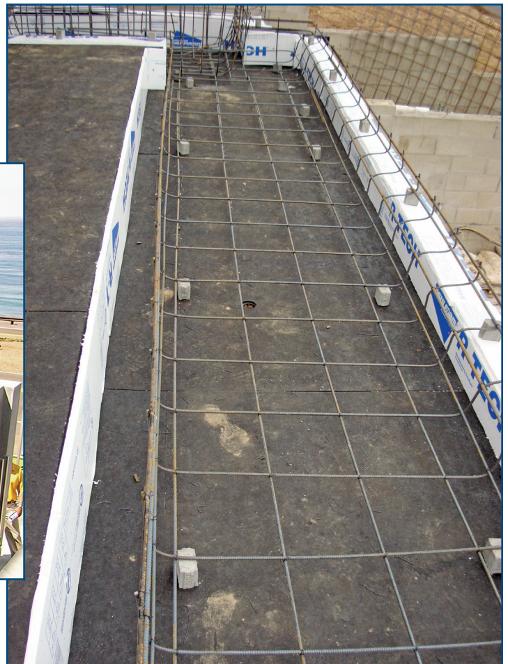
Figure 9 – Geotextile drainage composite laid flat.
